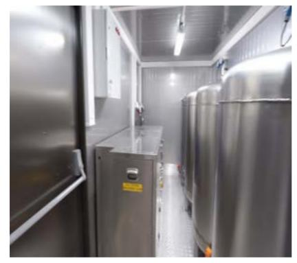
The system is equipped to work in all kinds of natural water resources. A pump and pump group that can draw water from water resources and pump purified water into water tanks. It has a treatment system with UV (ultraviolet) and reverse osmosis. A single-winged external door is located on one of the long sides of the 20 foot container. There is a diesel generator. Mobile water analysis can be done with the water analysis set.
