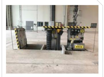
They are systems that provide the necessary energy and conditioned air for aircraft in maintenance hangars.
