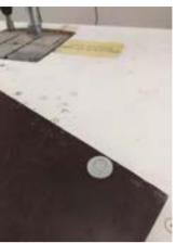
Dummy panels, which replaced the floor panels removed for maintenance, slide when the personnel walks on them. As a solution to this problem, panels containing vacuum rubber shoes that trap air inside have been produced.
